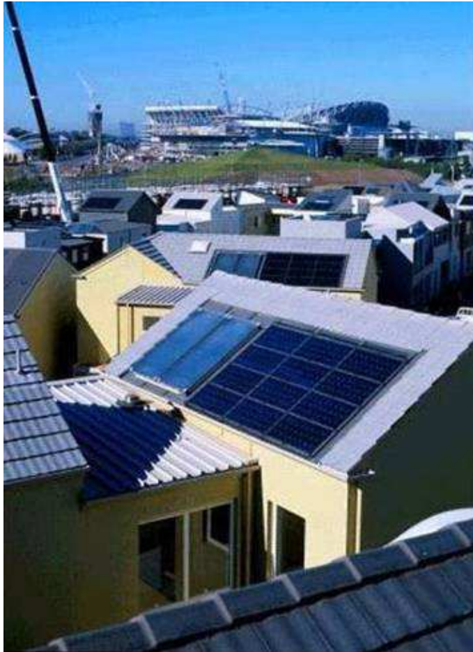
Solar powered suburb of Newington – former Sydney Olympic 2000 village
